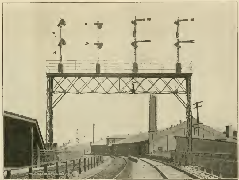
SIGNAL BRIDGE AT NEWARK, N. J., ON THE D. L. & W. TWO RIGHT HAND TOP SIGNALS HAVE EACH AN ELECTRIC SLOT MECHANISM. DWARF SIGNAL ON LOWER CHORD OF BRIDGE. BRIDGE MARKED C IN DIAGRAM.
